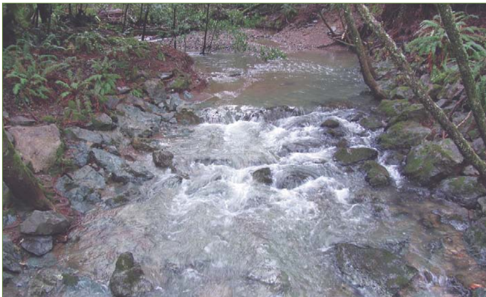
The Salmon Enhancement Project would remove many large boulders that stabilize the banks of Redwood Creek.
