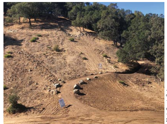
A portion of the Ponti Ridge Road-to-Trail conversion shows the steep former fireroad before (left) and the wider, multi-use trail after (right). Next step: erosion control and spreading native seed.
